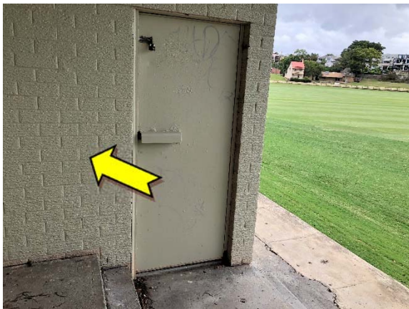
Photo 9. Exterior, shed, throughout, walls – suspected lead-containing beige upper coloured paint system.
